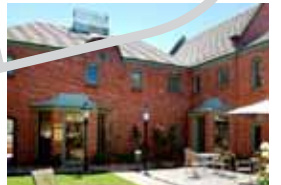
LEASEHOLD SERVICED APARTMENTS BALLART, VIC
